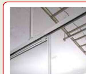
Hanging sliding doors with an opening of 2 m supported by upper and lower frames.
