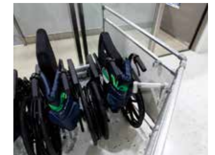
The fence for the wheelchair space uses a hinge connector at the corner, and its specifications enable it to open and expand the space.
