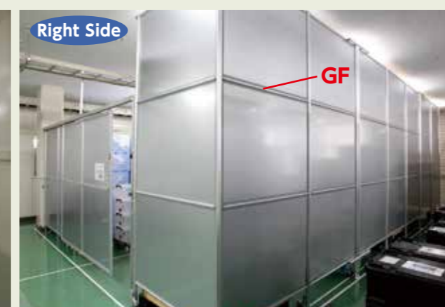
In order to carry in and out material from the back shutter, casters were attached to all the foot suspensions, making it movable.
